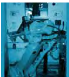
Compressed air pipe systems, vacuum pipe systems for automation
